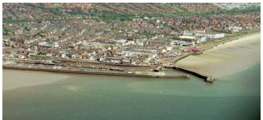
Harbour and Docking facilities
