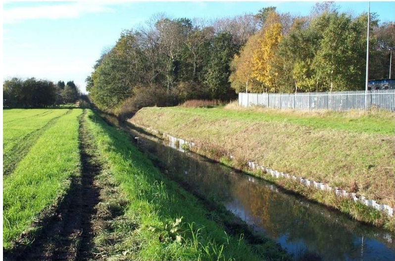
Typical piled drainage channel
