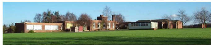
Burton upon Stather Primary School - Rear view
