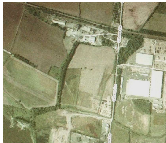
Transwaste Melton (Under construction)
